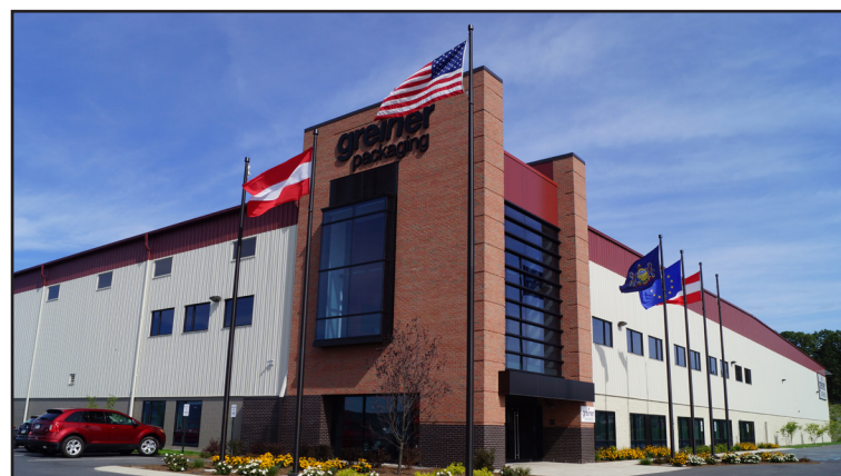
Greiner Packaging operates out of this state-of-the-art facility in Pittston, PA.
